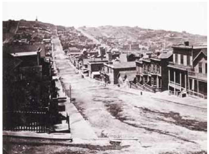
The block of Green Street on which the Seligmans and Rogers brothers lived, looking west from Kearny, 1860–1870.
